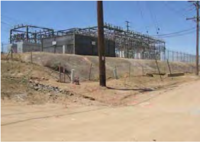
Illustration 1. Creelman Substation facing west.
