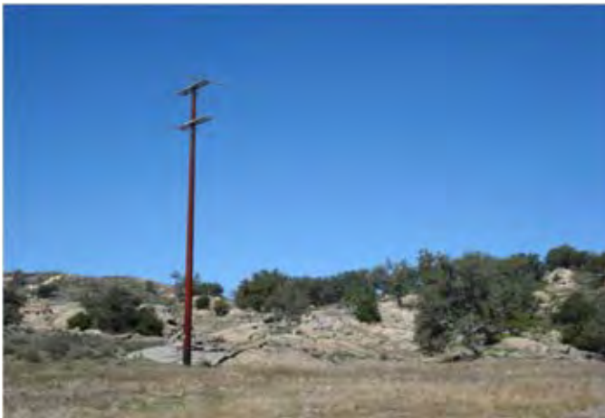
Illustration 14. View of TL 637 facing north.
