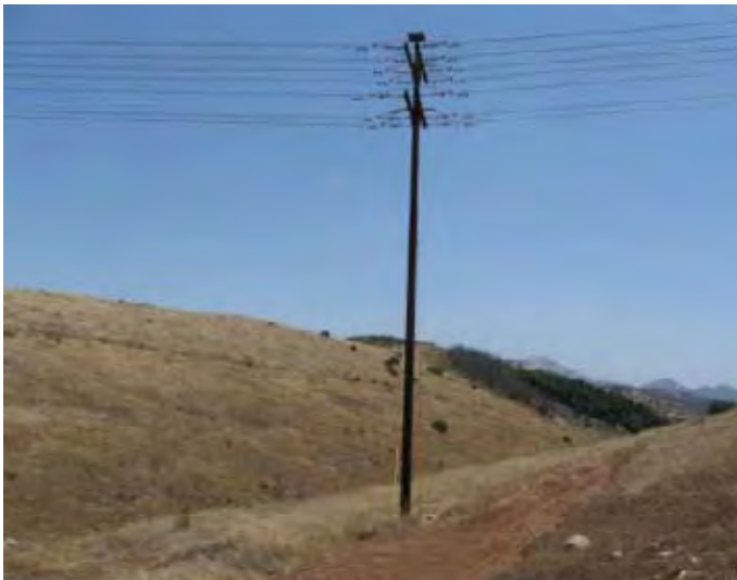
Illustration 2. Pole D28 facing north.
