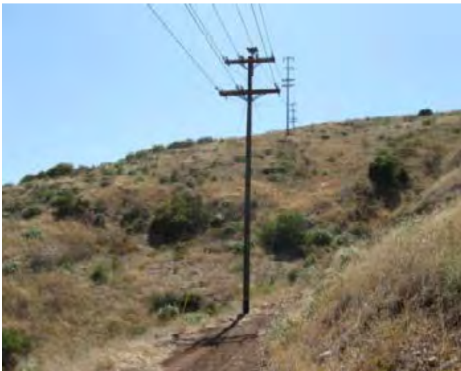
Illustration 3. Pole D31 facing northwest.
